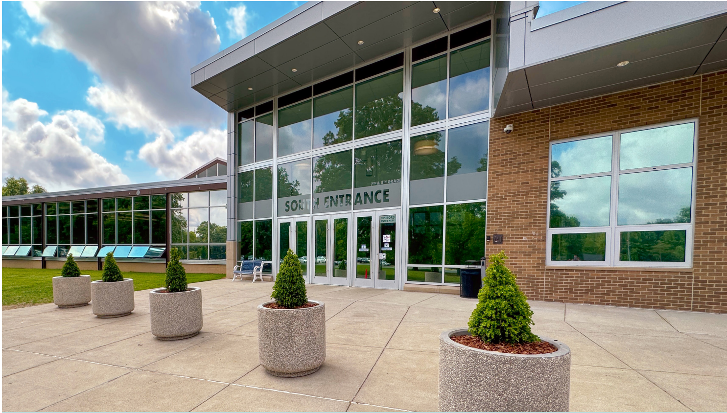
Entrance to WCMS with security bollards in place
